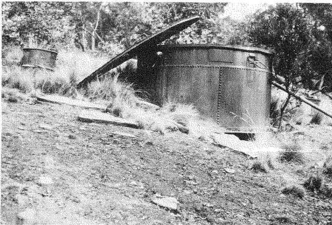
Fig. 5: Still No. 2, showing lid resting on the tank, the chimney to the left, and the hearth and condenser pipe to the right.
